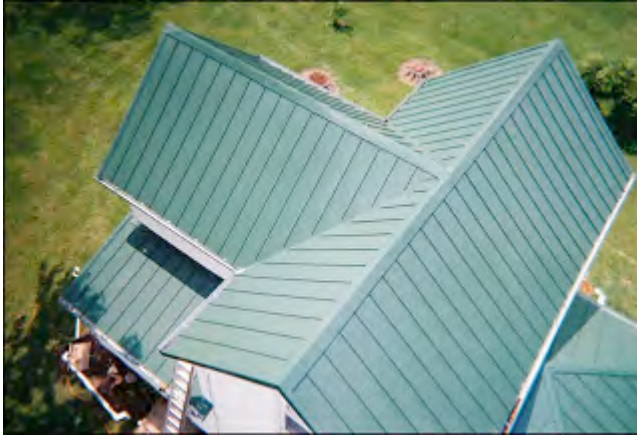
Figure 7: A Typical Residential Roof
