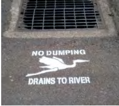
Figure 11: Spray Paint Marking
