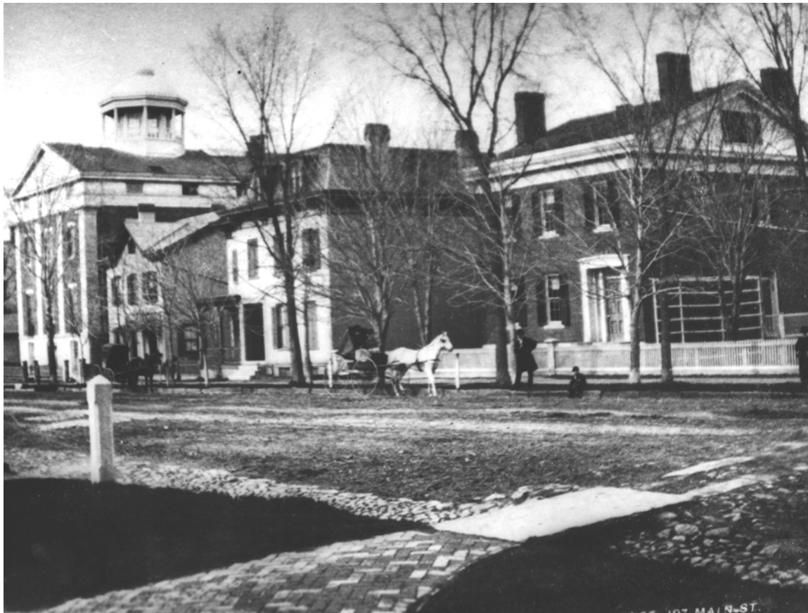
A historic photograph of Geneva's South Main Street shows permeable pavers, street trees and a bio-swale.
