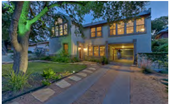
Figure 2: Small Stone Driveway
