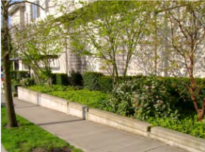
Figure 4: Example of Stormwater Planter
