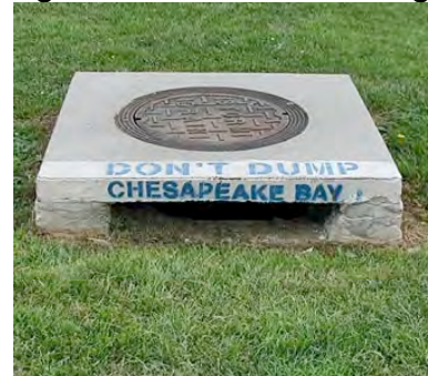
Figure 5: Storm drain marking
