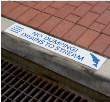
Figure 3: Storm drain marking
